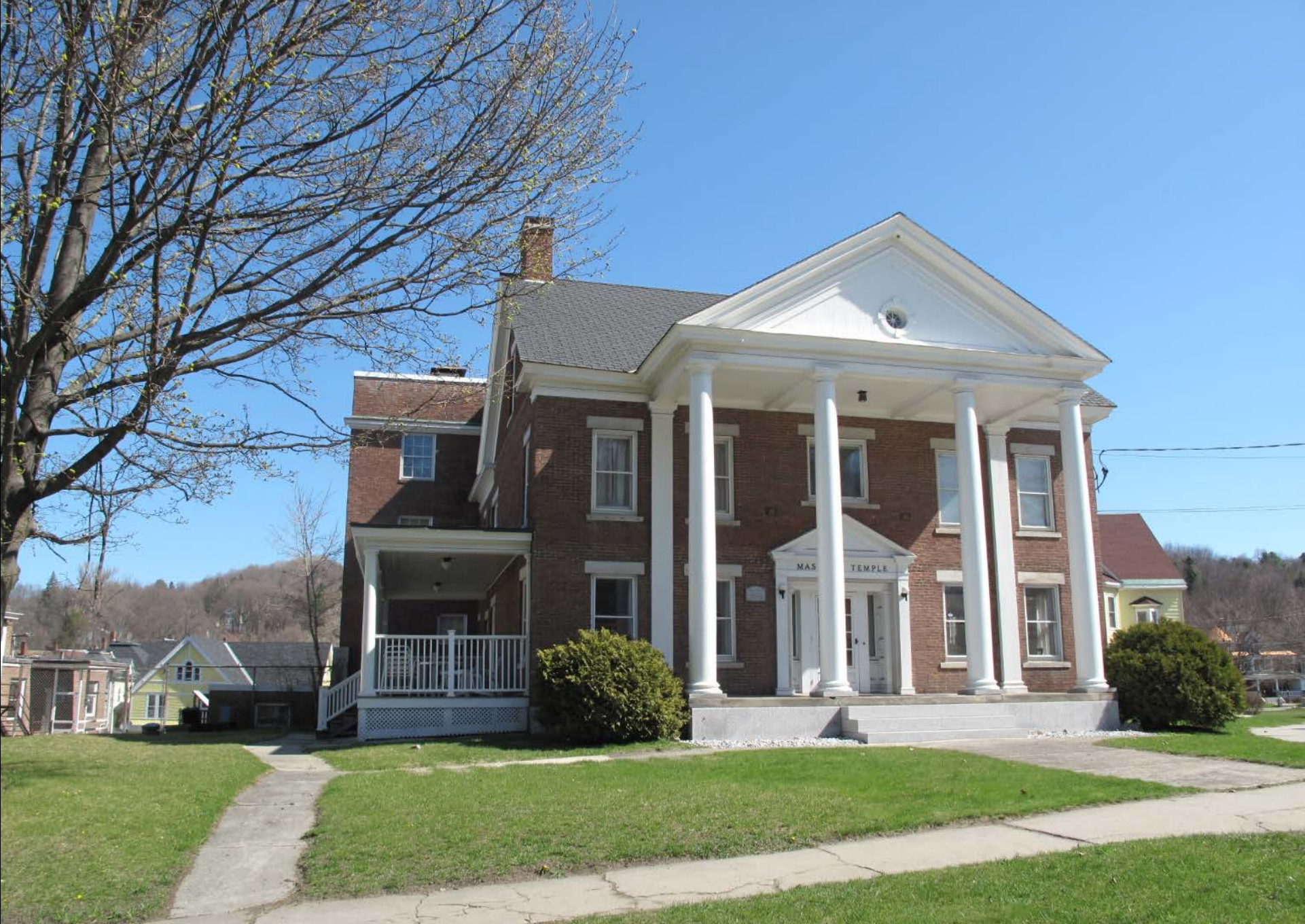
Photograph 16: View looking northeast at Masonic Temple, façade, HD # 8
