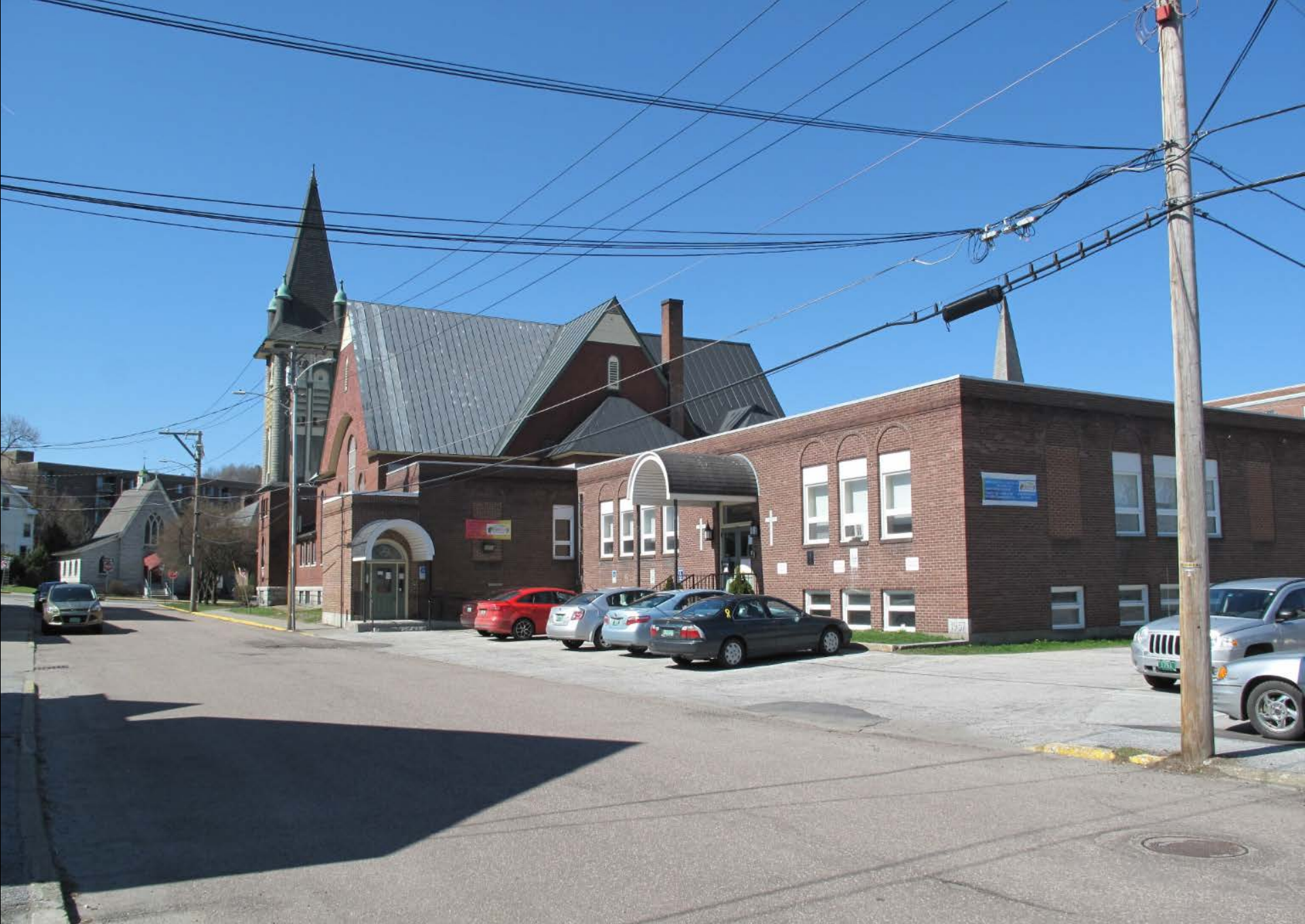
Photograph 12: View looking southwest at Hedding Methodist Church, rear addition, HD #6
