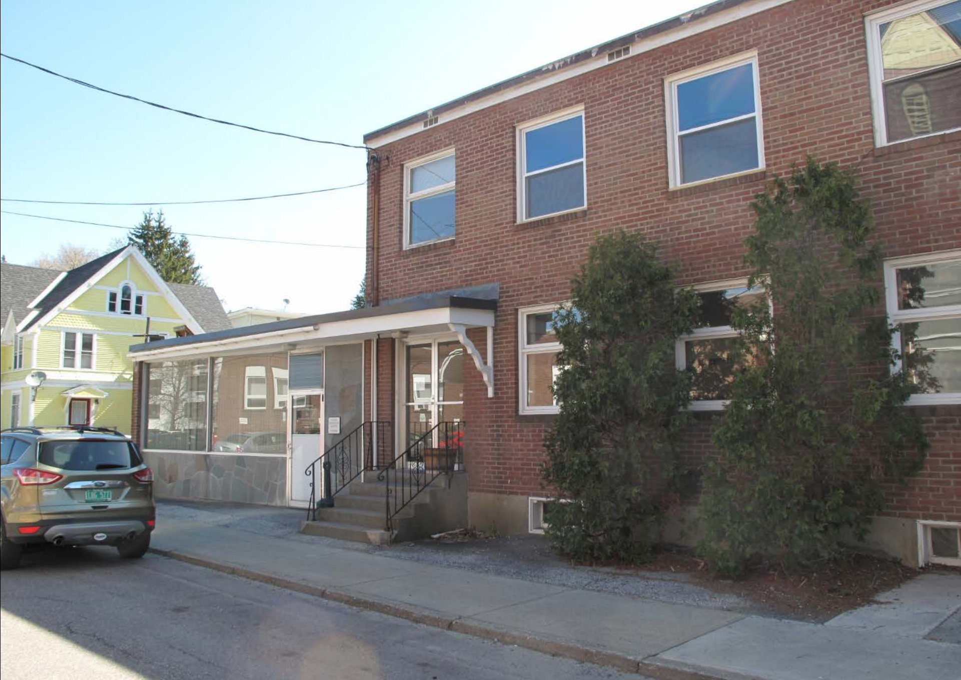
Photograph 15: View looking northeast at Apartment Building, rear addition, HD #7
