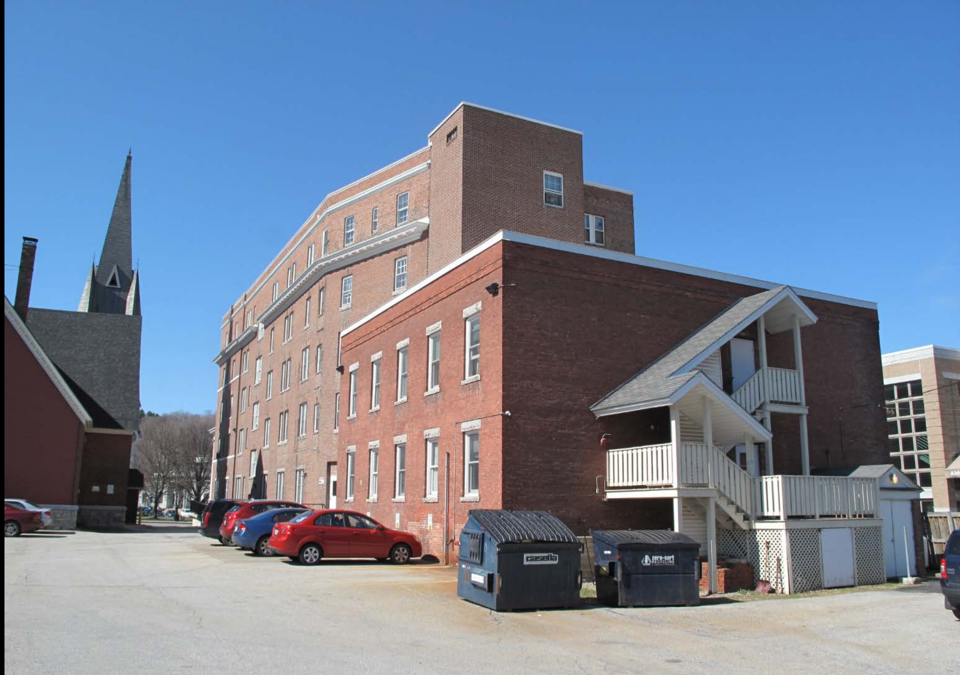
Photograph 8: View looking southwest at Hotel Barre/Washington Apartments, south elevation and rear addition, HD #3
