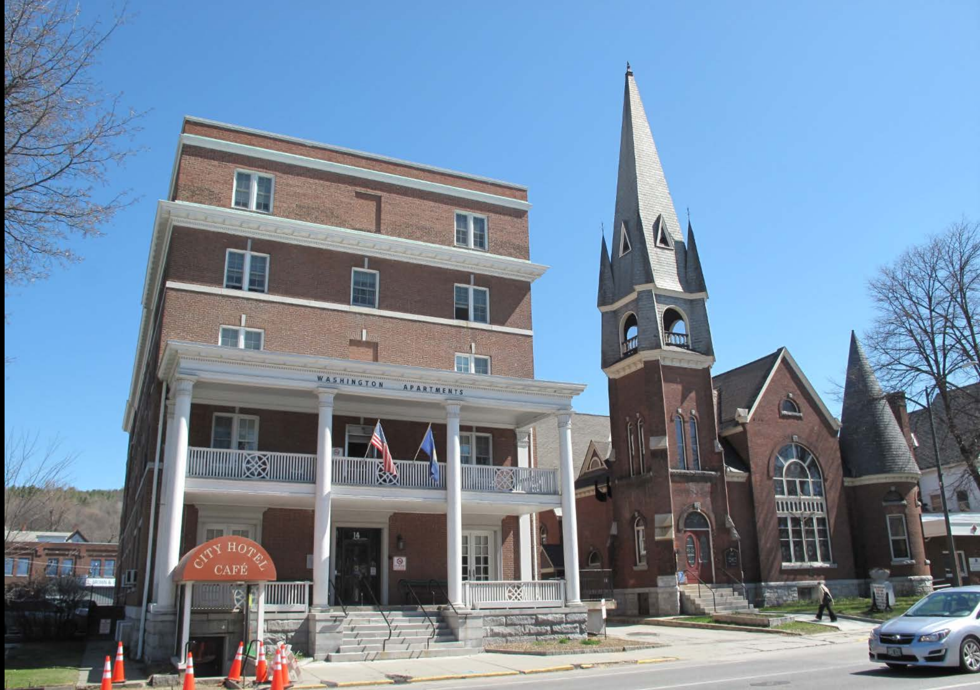
Photograph 7: View looking northeast at Hotel Barre/Washington Apartments (left), HD #3, and First Baptist Church (right), HD #4
