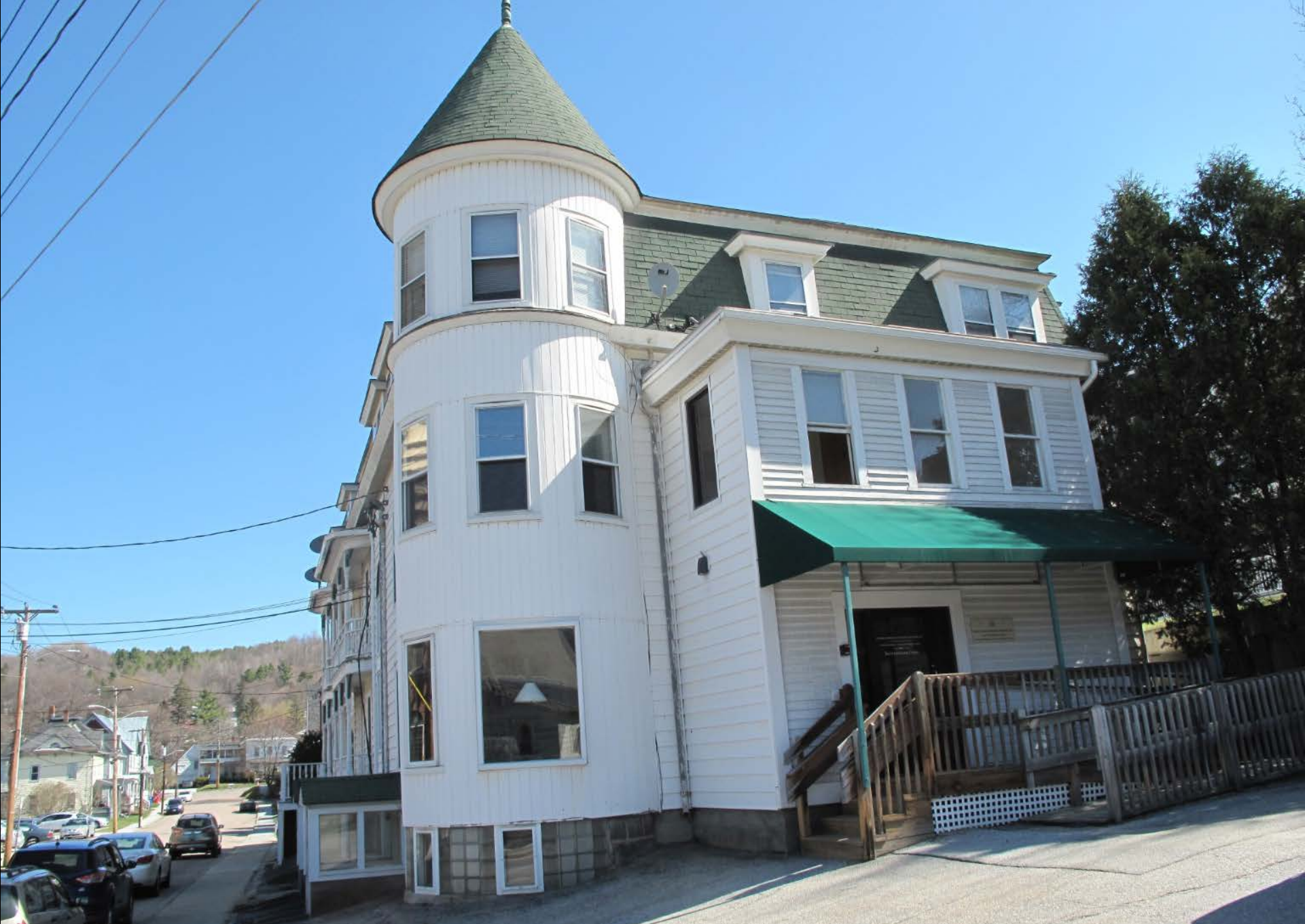
Photograph 14: View looking northeast at Apartment Building, façade, HD #7
