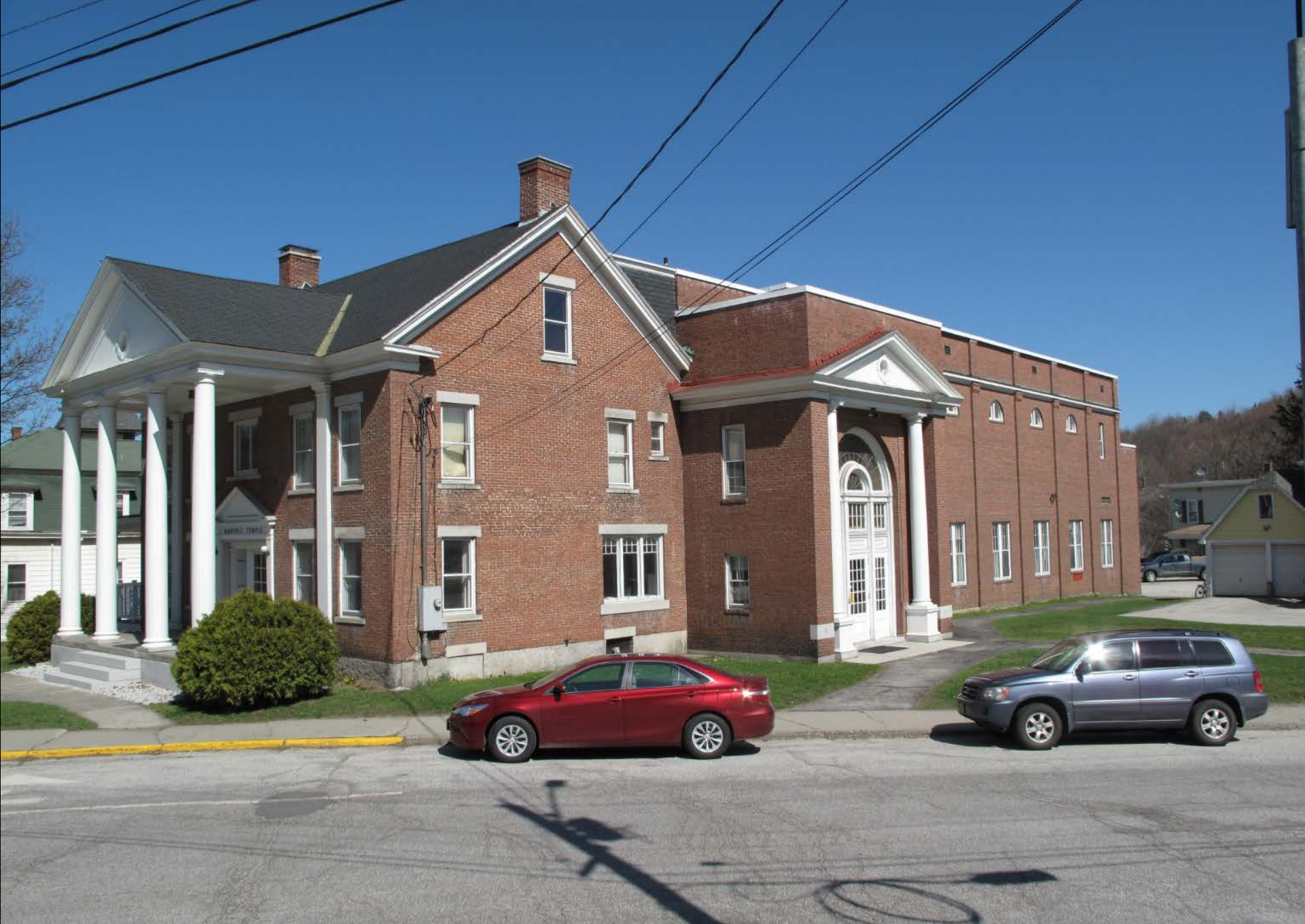
Photograph 17: View looking north at Masonic Temple, rear addition, HD #8
